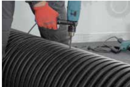
3. Drilling holes for the guided crown saw
