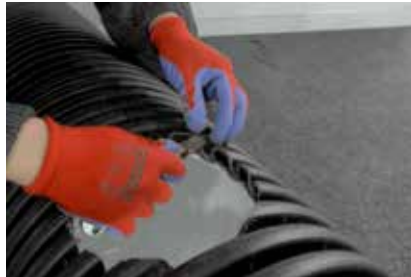
5. Cleaning chips and forming a clear hole
