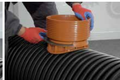
12. Final tightening of sag
