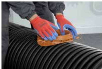
9. Tightening the sag
