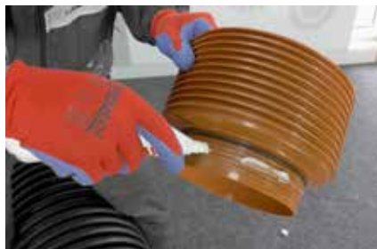
10. Lubricating appropriate connection of sag
