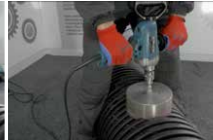
4. Drilling holes with crown saw
